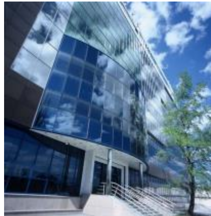
Parkur Tower, Warsaw
